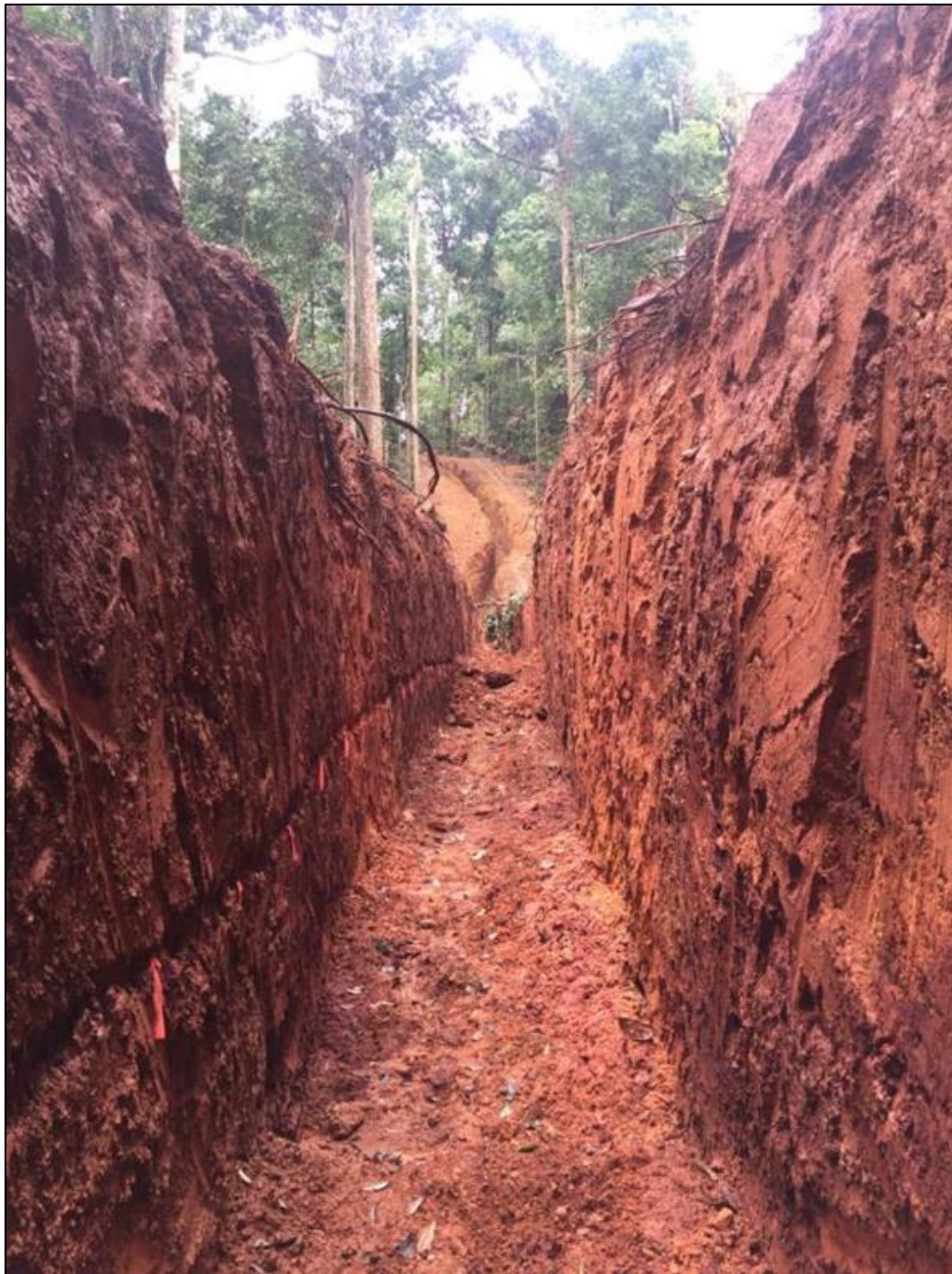
Figure 9-3: Salbora trench TRSB18-002 – horizontal sampling channel in left-hand wall Source: Goldsource (2018)
